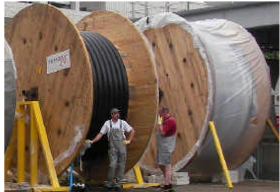
Figure 3: Flexible transfer lines delivered to NSRRC and the supporting frame to unroll these lines.
